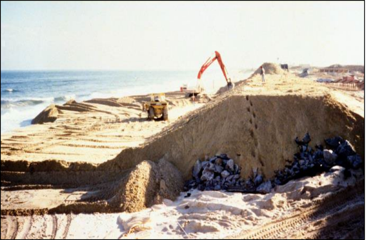
FIGURE 9.—Construction of a composite seawall in Virginia. Illustration credit: USACE (2018a).
